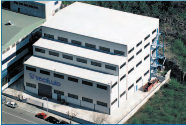
R+D, Manufacturing and assembly workshop
