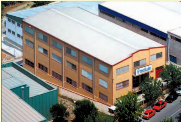
Sales department and calibration facilities
