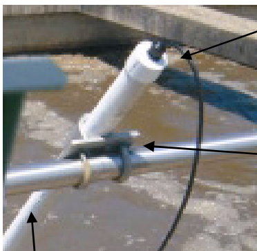
Probe Held in Position by 40mm (1.1/2") Pipe
