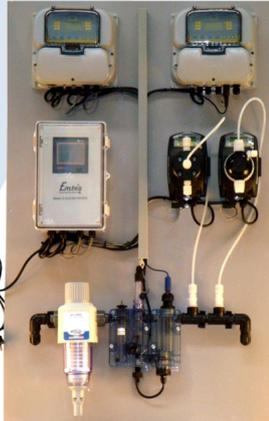
**Chlorine Dosing and pH Correction with Data Logging**
