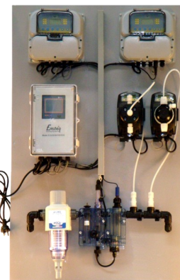
Chlorine Dosing & pH Correction with Data Logging
