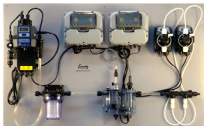
Chlorine Dosing & pH Correction with Turbidity Monitoring
