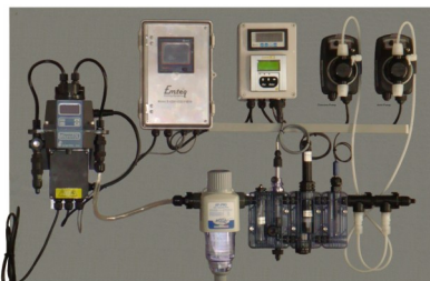
Chlorine Dioxide Dosing, pH Neutralisation Turbidity Monitoring with Recording & Data Logging
