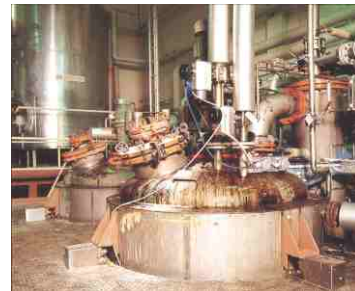
Batching Processes Reactors and Process Vessels
